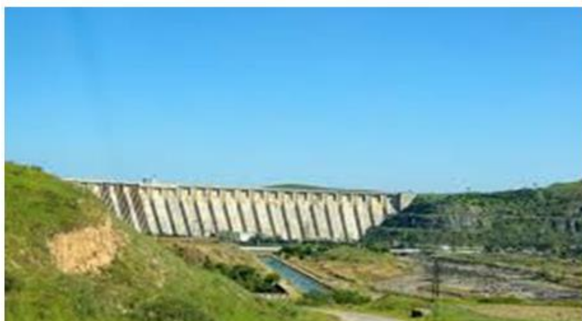
Fig. 1. Dam of the Karkidon reservoir
